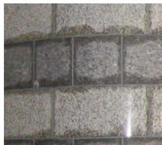
Staining on polished granite. Unknown age.
