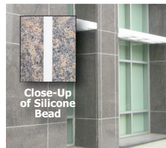
No staining or dirt pick-up on Cold Spring Carnelian granite after four years.
