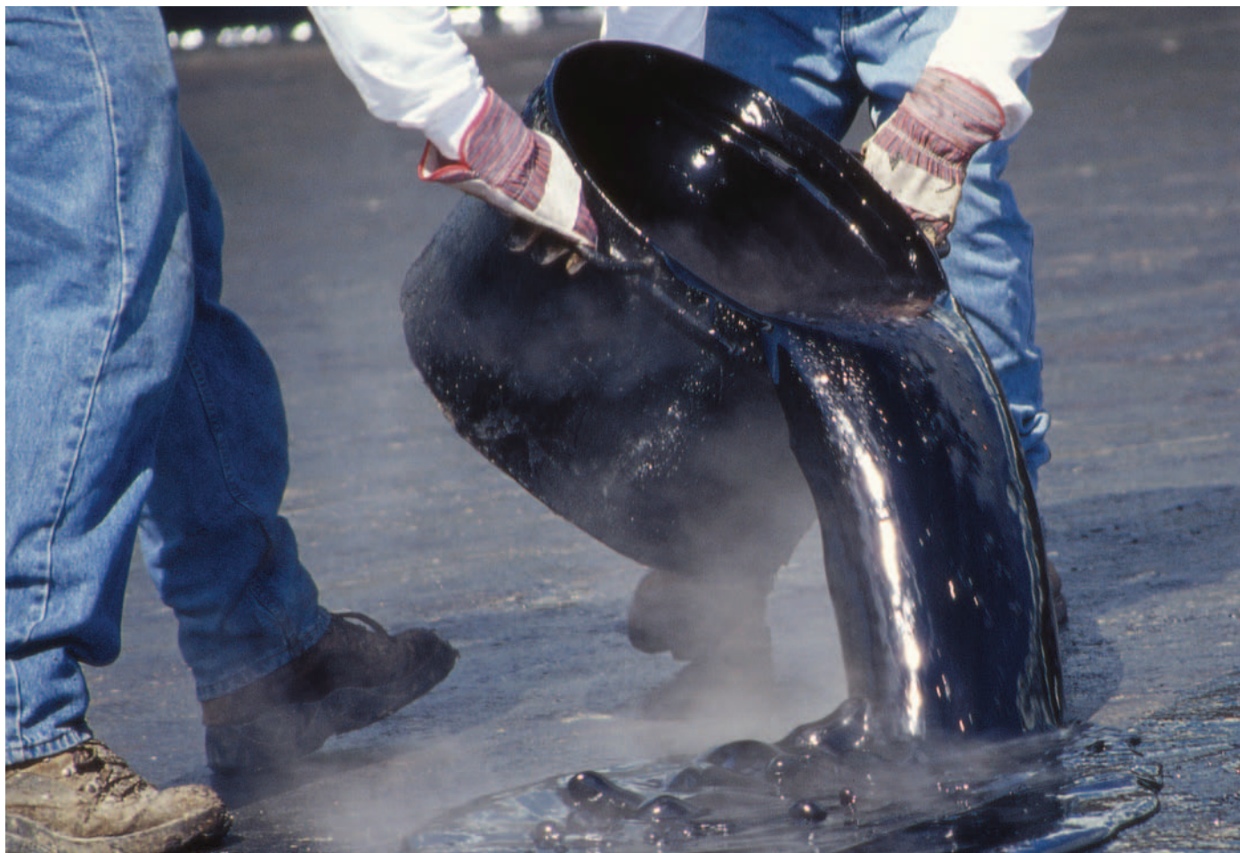
CCW-500 application to a roof deck.
